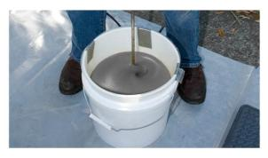
3. Recommended ratio of (4) liters of FORTRESS to (4) kilos of ordinary Portland Cement (OPC). Make sure that the cement has been thoroughly sifted. Pour the FORTRESS in a clean container. Gradually add ordinary Portland Cement (OPC) while constantly mixing. Continuously mix from 5 minutes to 10 minutes. For electric mixing, recommended 5 minutes minimum. For manual mixing recommended 10 minutes minimum.
